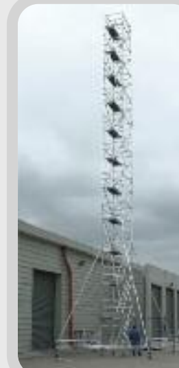
Test build of a 20m free-standing mobile tower at the Instant UpRight factory in Dublin, Ireland.
