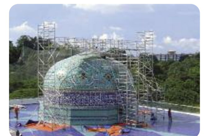
Pool Bridge Scaffold and Cantilever Towers at the mosque in the Kuala Lumpur Federal Government Building, Malaysia.
