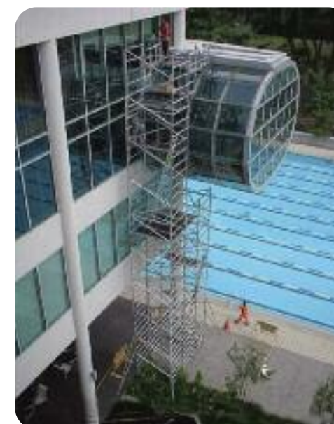
Test build of a 20m free-standing mobile tower at the Instant UpRight factory in Dublin, Ireland.
