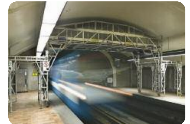
Special Rolling Bridge for Metro Station roof maintenance.
