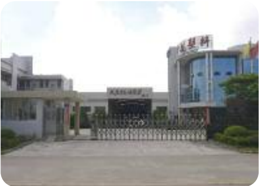
Instant UpRight International Manufacturing Plant, Guangzhou, China.
