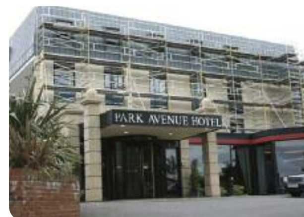
Aluminium Façade Scaffold - Park Avenue Hotel, Belfast.
