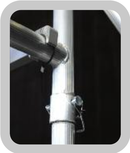
Brace Hook Frame Locking Pin
