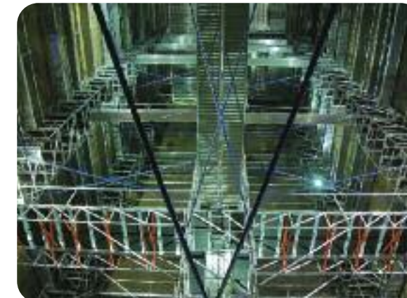
Quick-Erect Boiler Scaffold System at Manjung, Malaysia. View looking from the bottom of the hopper showing the outer support trusses and main tower structure. The boiler scaffold for this 660MW unit was commissioned in 2007.
